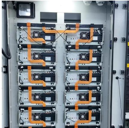
A battery rack cabinet is a specialized enclosure designed to securely house multiple batteries in energy storage systems. It ensures thermal management, safety, and scalability for industries ...
